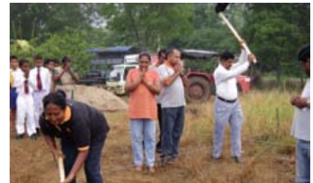
Foundation laying Buttala Suboda School development Project
